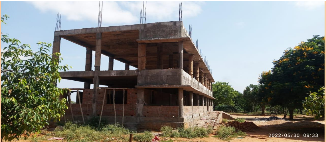
Construction of New Classrooms Block
